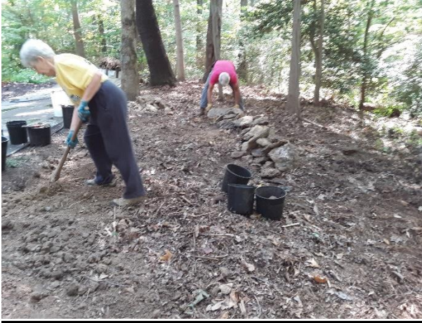
Carolyn Beck quarries rock and Lars Larson "builds" a wall
